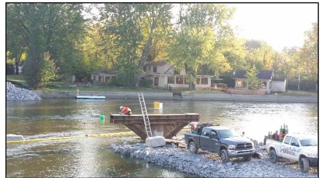
Once the first support beam and "T" was in place, they began digging out the rocks, putting them in a dump truck, and driving them to the other side of the river. Here's a photo of that process. You can see how the "T" is left behind as they take out the rock access.
