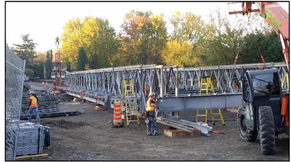
Once the post was driven in far enough, they filled it with concrete. You can see the post in the photo. In addition, you can see that they have pushed the bridge structure well past the north support beam – getting ready to join up with the south part of the bridge.
